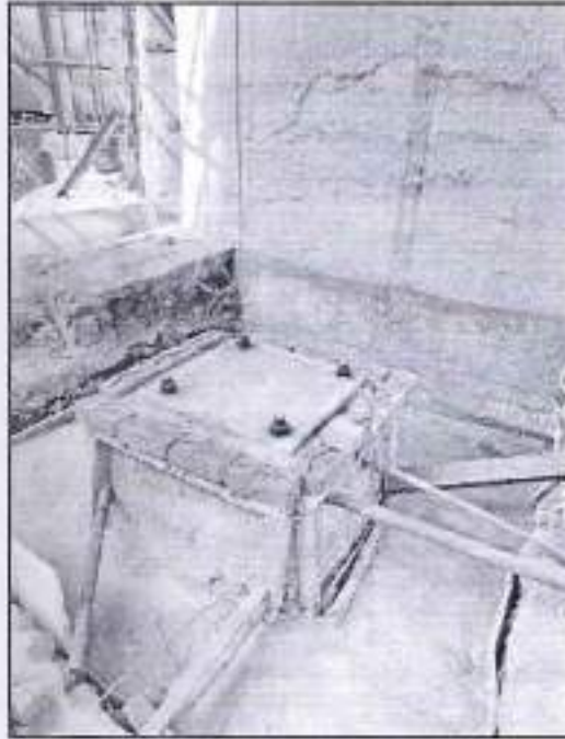
Kundarkhi – Foundation Work
