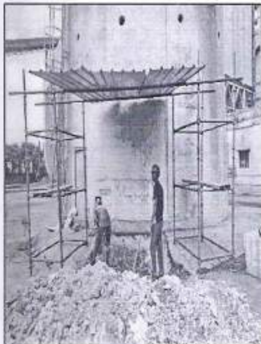
Utraula – Foundation Work
