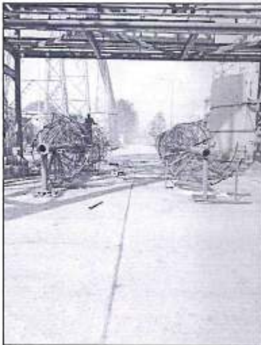
Khambarkhera – Fabrication Work
