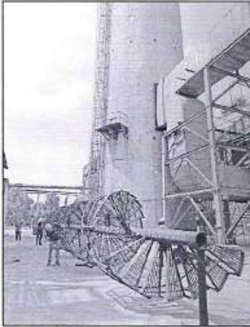
Maqsoodapur – Fabrication Work
