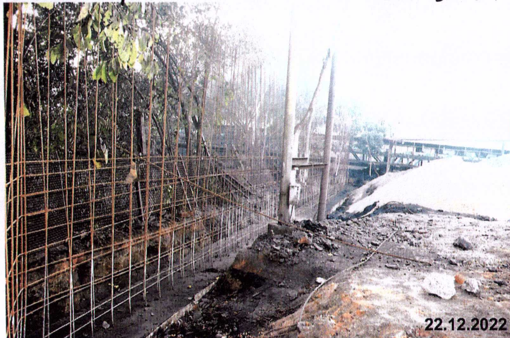
CONSTRUCTION WORK IN PROGRESS OF BOUNDARY WALL
