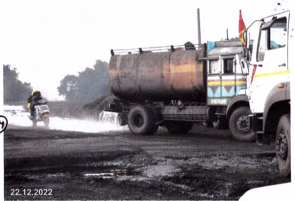
Mobile water Tanker sprinkly water around Project Area.
