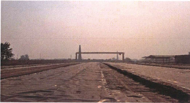
RMS Area with Overhead Crane Actual Image
