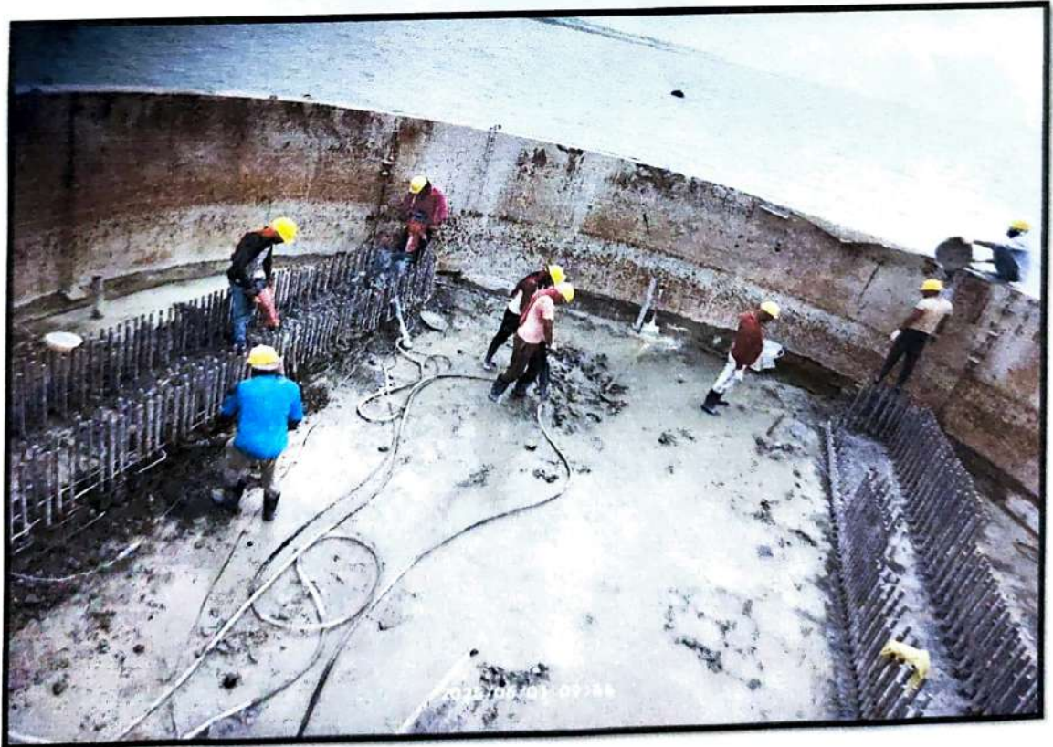
P11 Pier shaft removal completed on 01.06.2025
