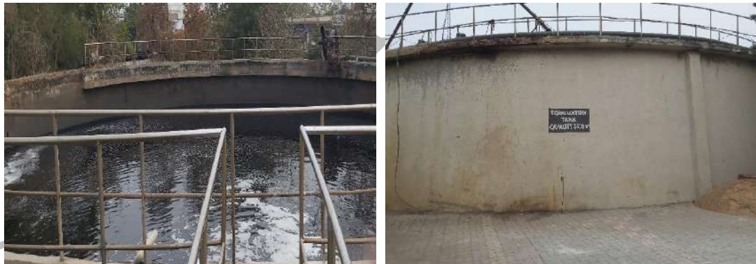
Figure 9.4: Collection cum equalisation Tank with intermittent mixing
