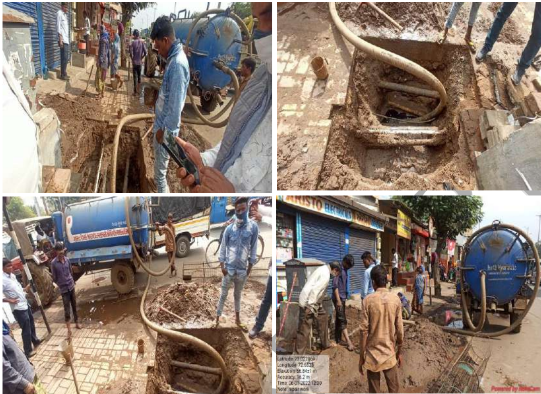
Figure 8.2: Repairing of leakage work in Mega Pipeline
