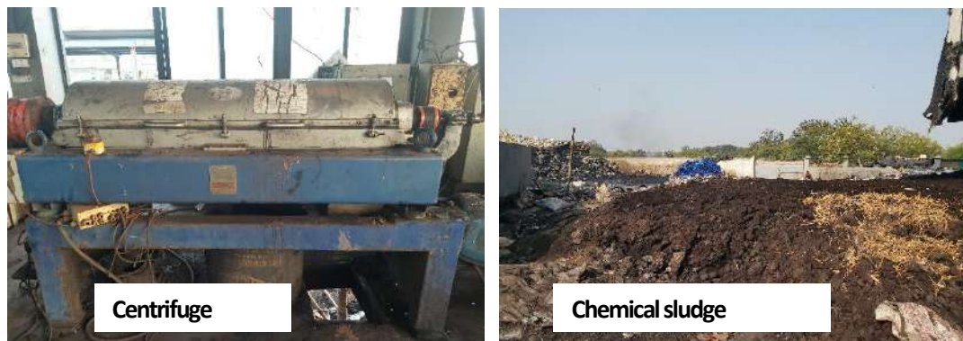
Figure 7.7: Centrifuge and dewatered chemical sludge laying within the CETP premises
