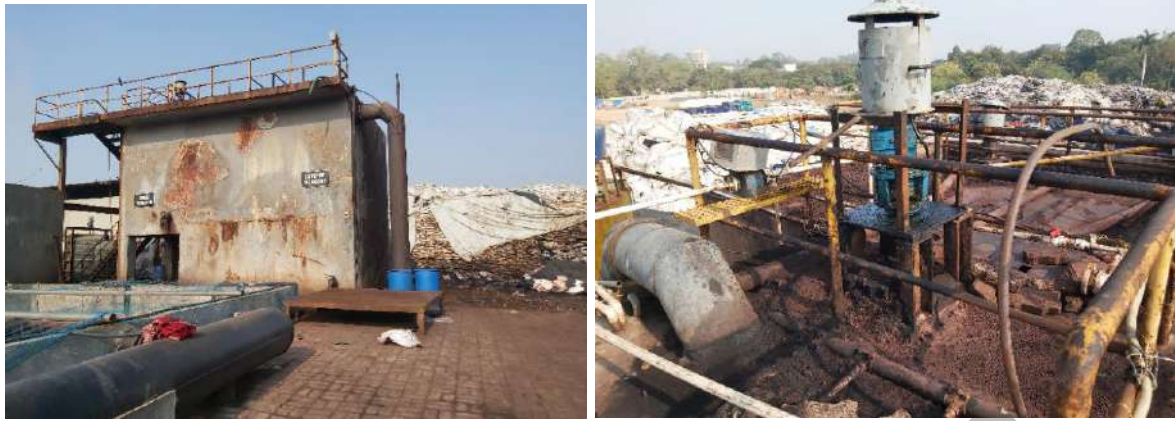
Figure 7.11: Existing condition of post treatment units
