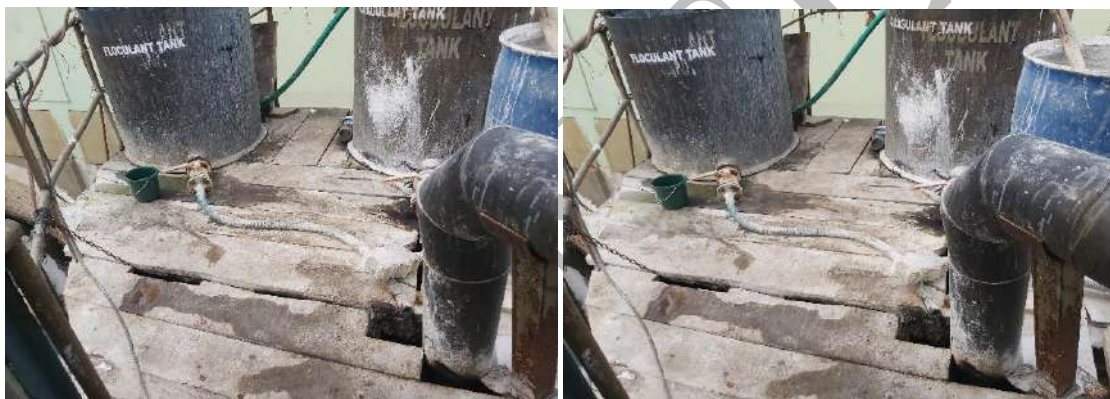
Figure 9.6: Addition of coagulants in flash mixer with NO Agitation
