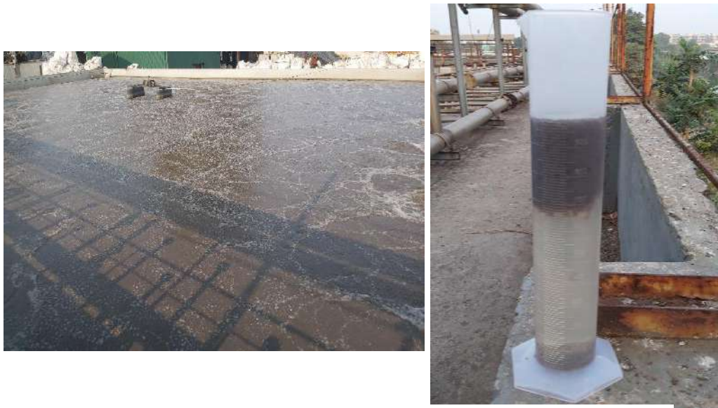
Figure 7.16: Biomass floated/bulked in aeration tank
