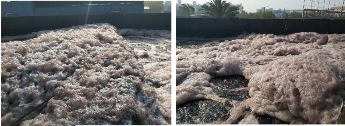
Figure 7.9: Massive layer of foam form in ACT – I
