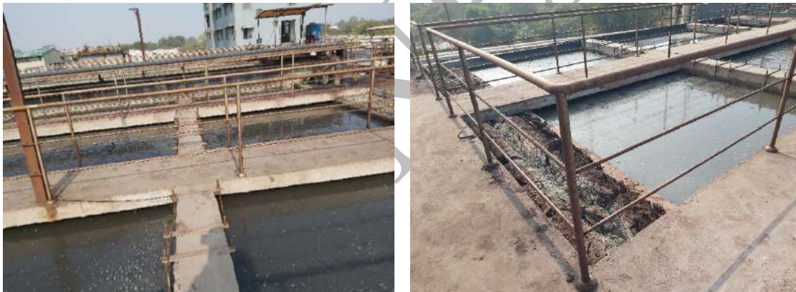
Figure 7.15: Formation of gas bubble in tube settler-I
