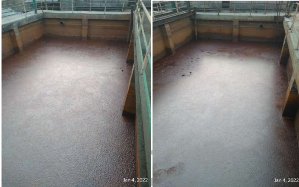
Figure 5.3: Additional effluent storage tanks outside CETP premises
