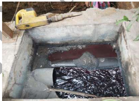
Figure 8.3: Non-mixed effluent routed to the aeration tank
