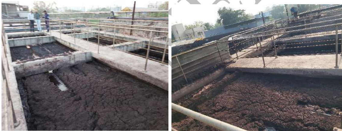
Figure 7.12: Chemical sludge fill in tube settler-II
