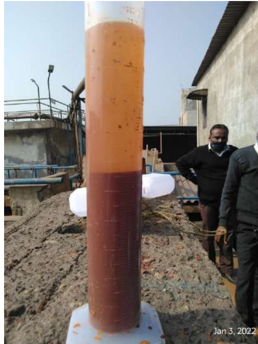
Figure 5.7: Excessive volume of inorganic solids in aeration tank 1
