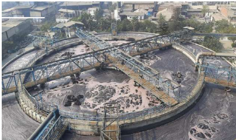
Figure 4.5: Counter-current circular aeration tanks with fixed & free aspirator type Surface Aerators
