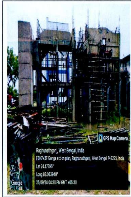
RAGHUNATHGUNJ STP SITE
