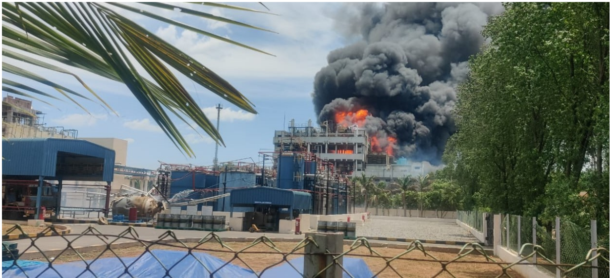
Fire broke out at SRS plant.
