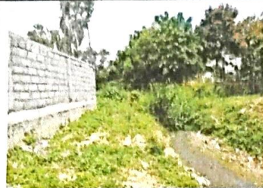
Compound exists in the nala buffer towards eastern side
