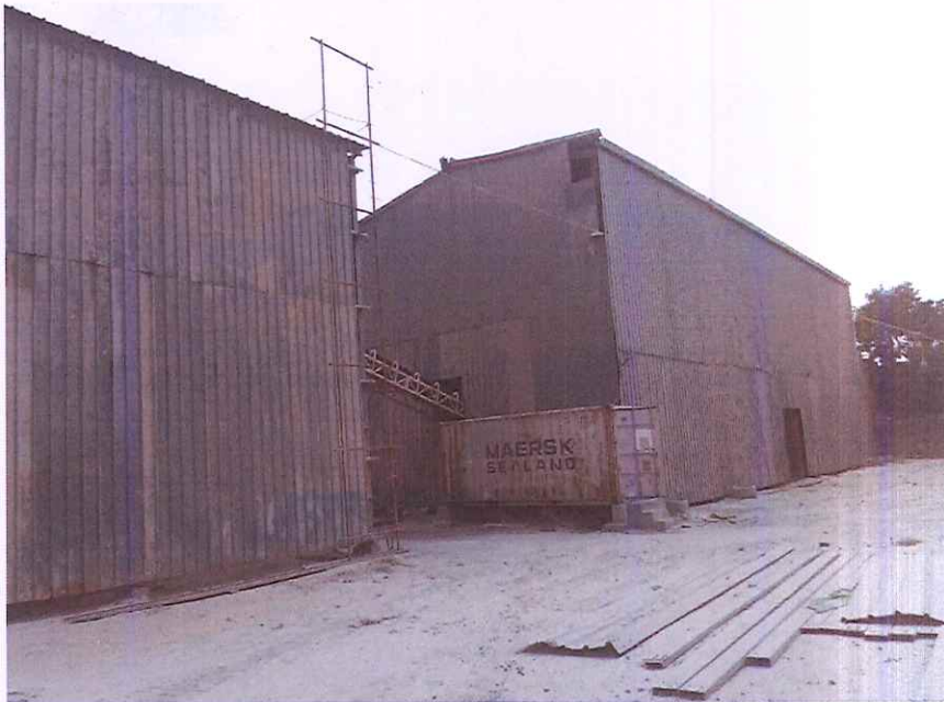
8 th respondent covered with GI sheet
