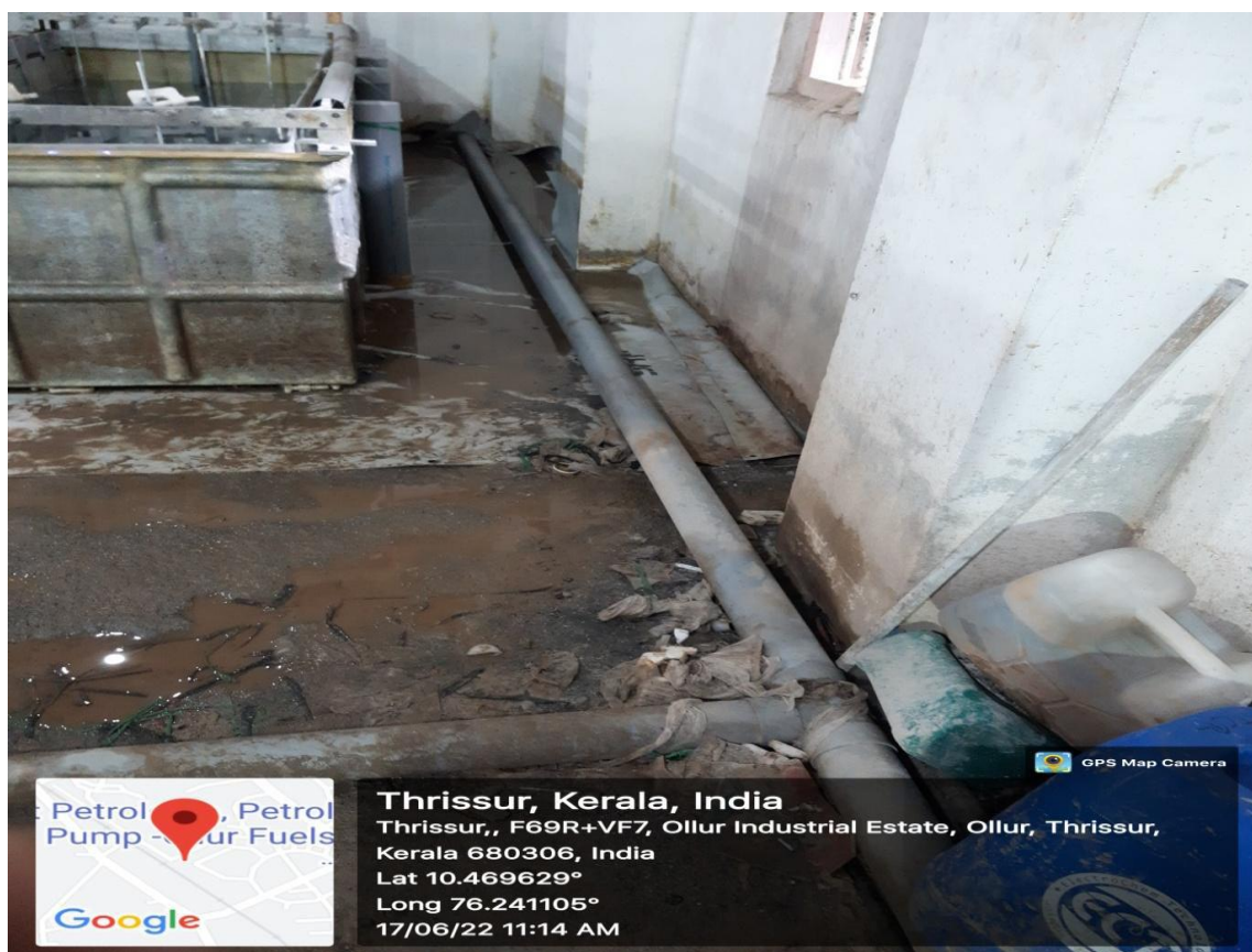
Figure 6 - Wastewater conveyed to the outside premises at Bright Precured Systems 2
