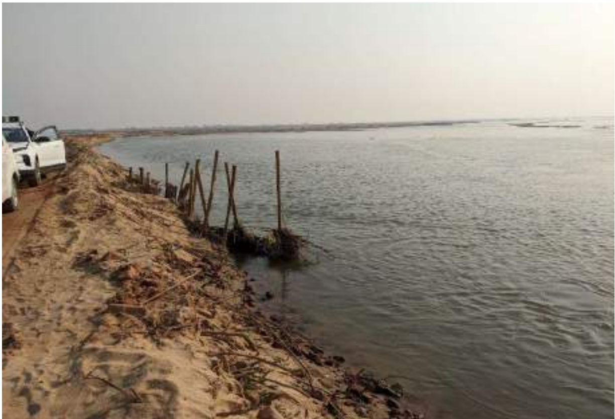
Pic 6: Extraction Path restricting and diverting the flow of river at Block No. 5
