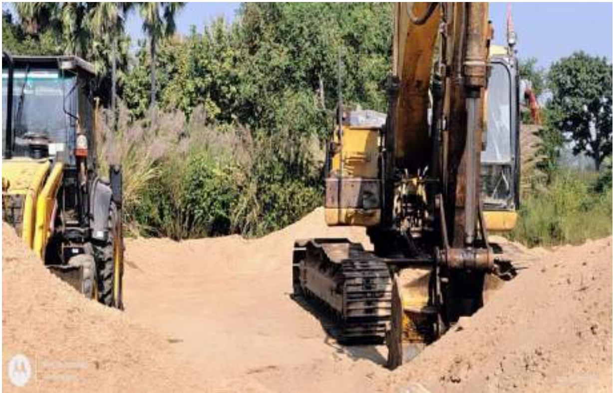
Pic 1: Excavator at Sand Block No. 1
