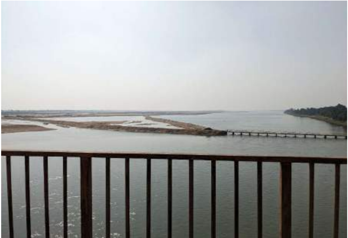
Pic 4: Extraction path at Sand Block No. 3A
