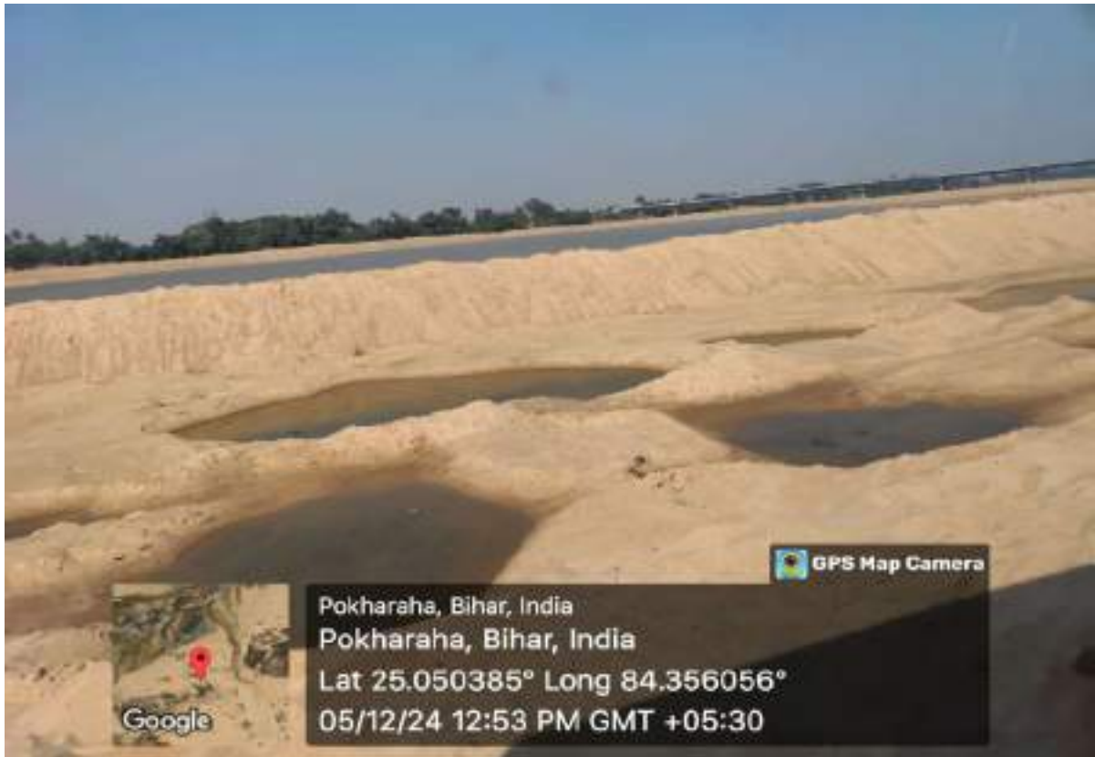
Pic 7: Enclosure of lease area with structure made of river sand at Block No. 6
