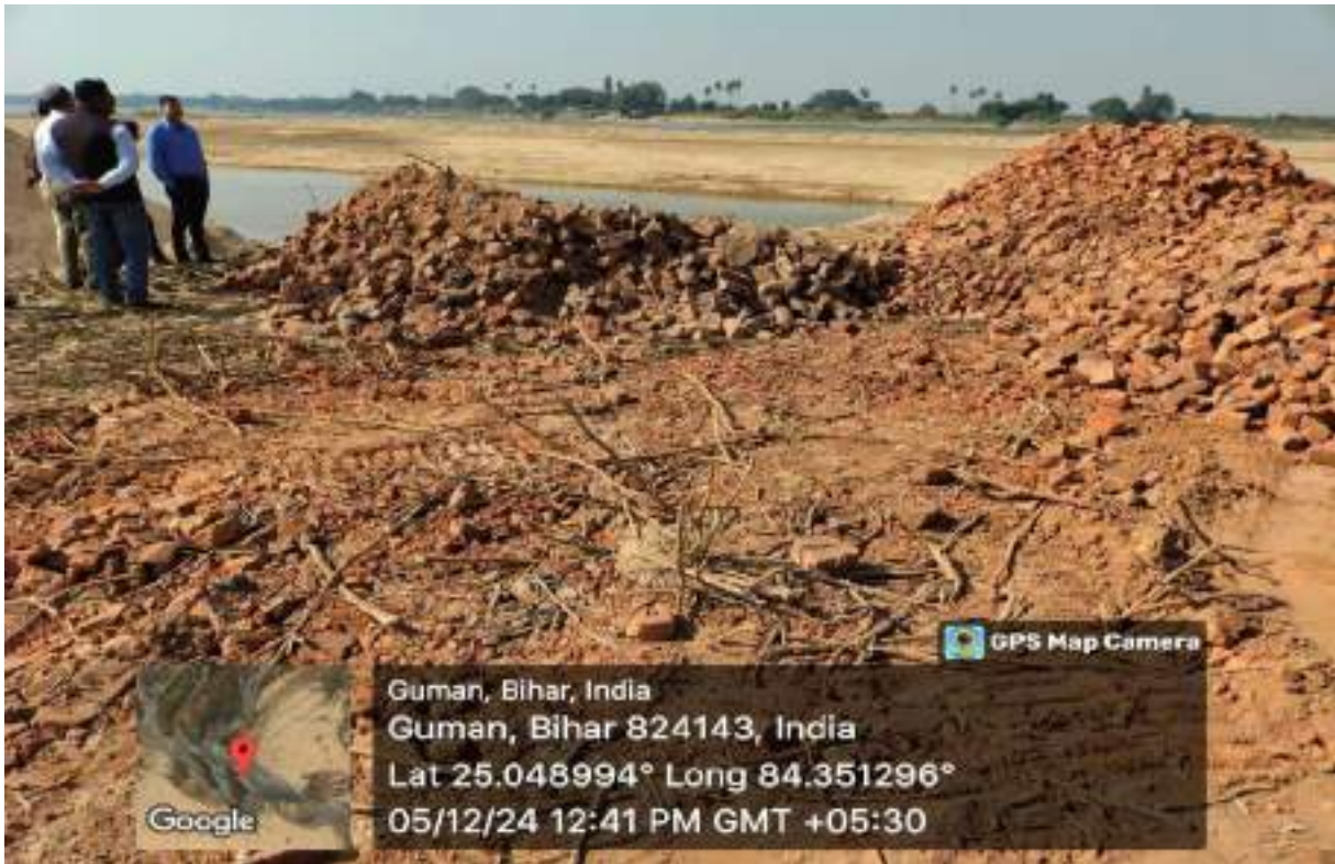
Pic 3: Brick bats and twigs used for extraction path making at Sand Block No. 3A
