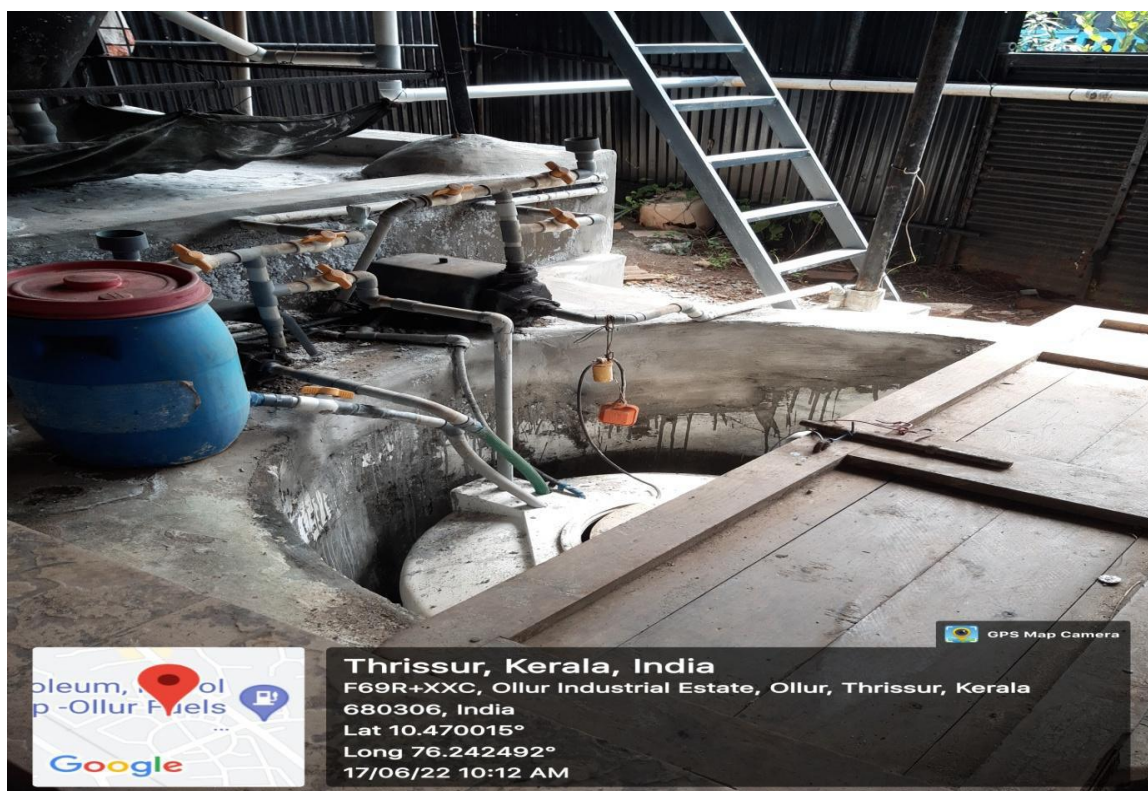
Figure 4 - Collection tank and chemical addition installations in ETP
