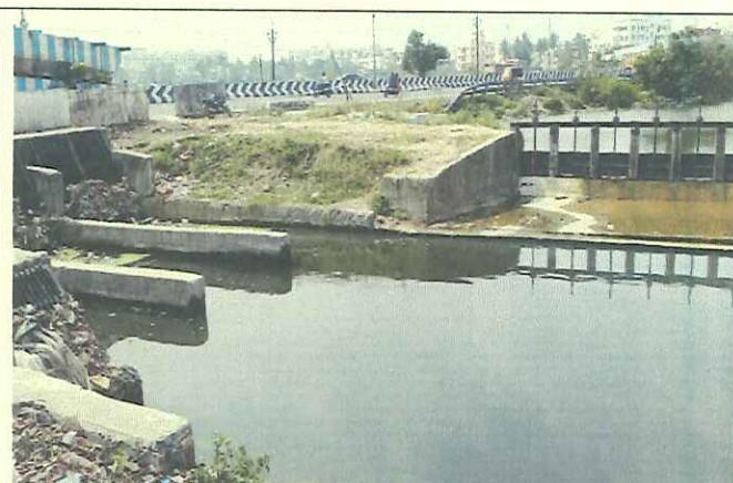
Cut and cover channel provided for the conveyance of the surplus water to the Pallikaranai Marsh Land
