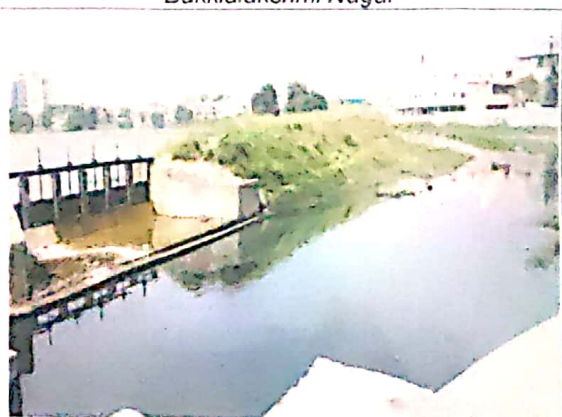
Surplus water from Narayanapuram Eri joining the surplus channel
