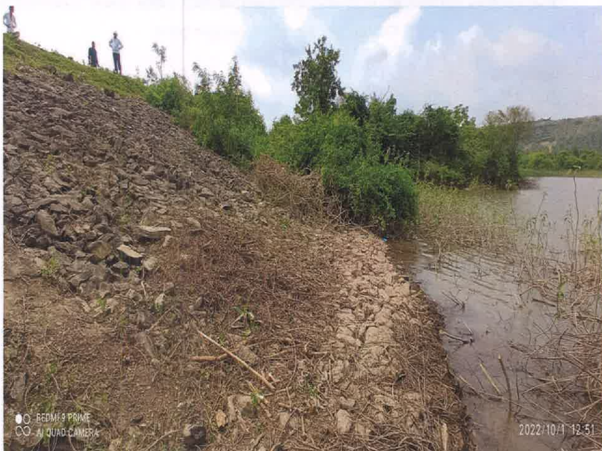
Earthen bund with stone pitching along Vattivagu reservoir
