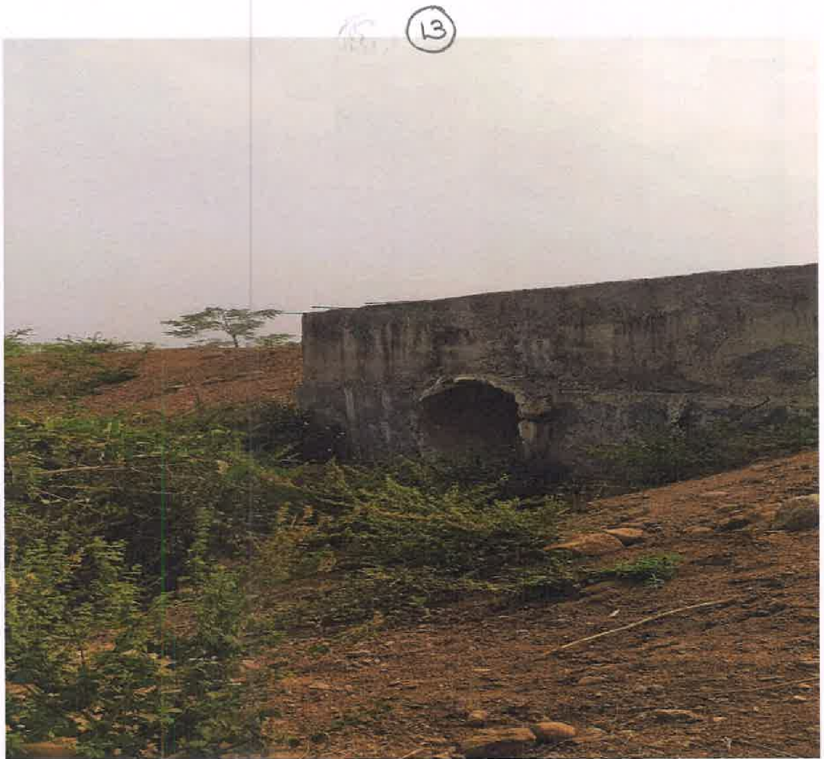
Hume pipe culvert constructed by SCCL in Ullipitta village
