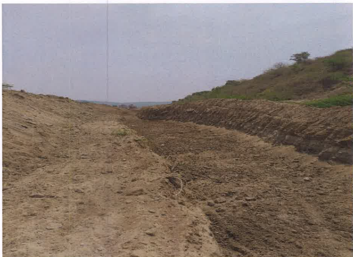
Deck drain at 1 st deck of D-3 Dump
