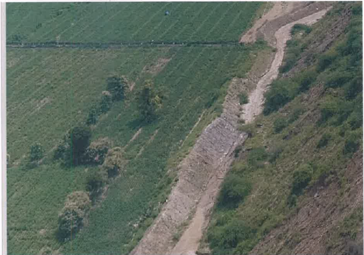
Earthen bund along D3 Dump towards Ullipitta side
