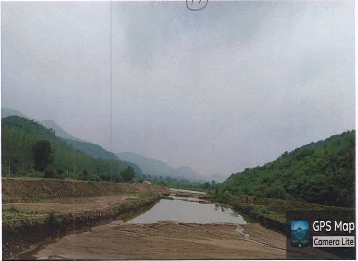
Three additional siltation ponds along D-3 dump
