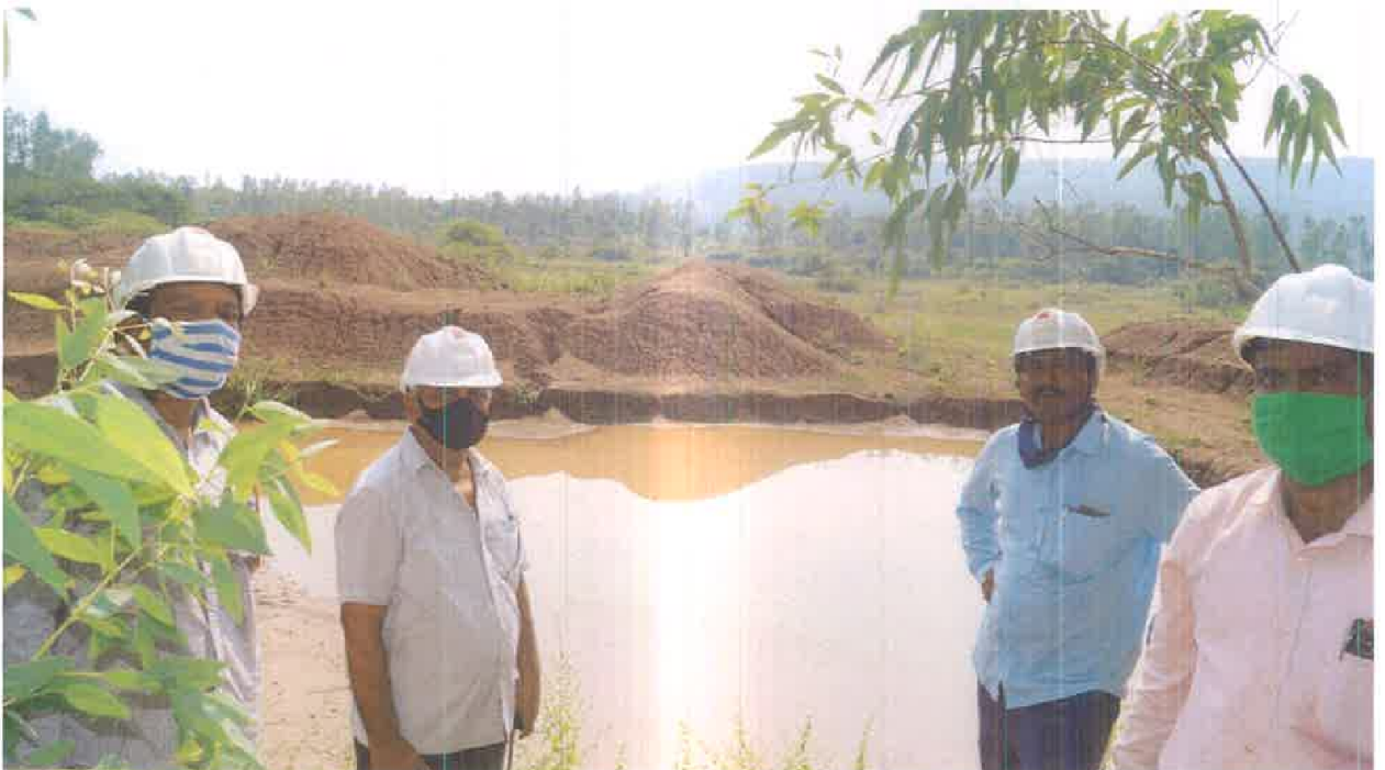
Settling pond beside D-2 Dump
