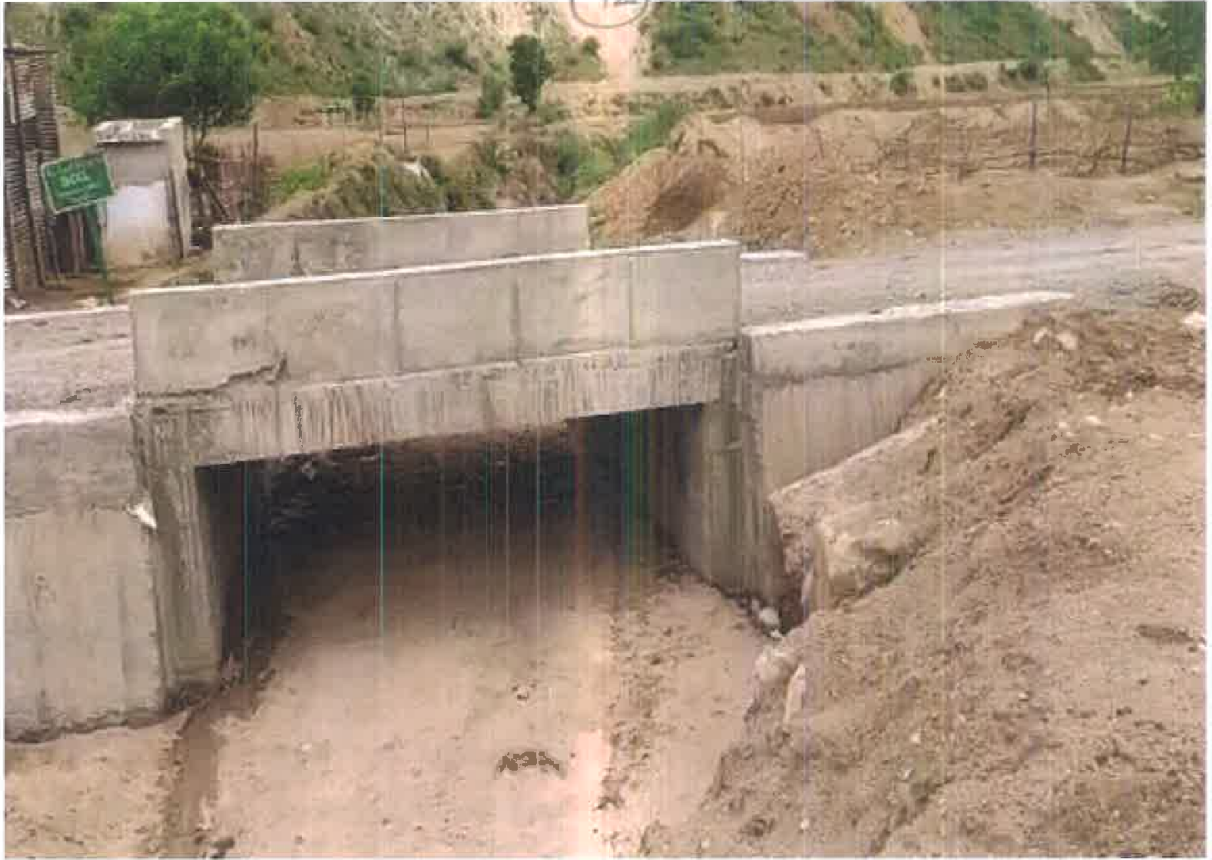
Box culvert constructed by SCCL in Ullipitta village
