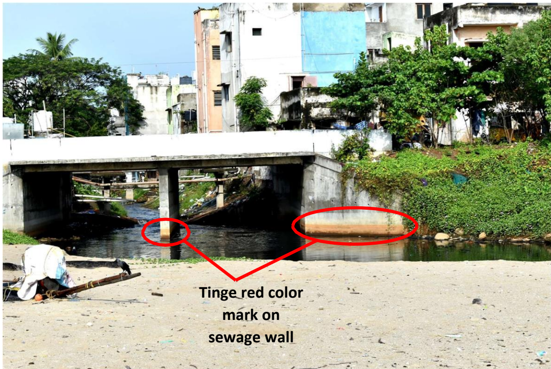
Fig 3: Persistent coloration on the walls of the sewage channel.
