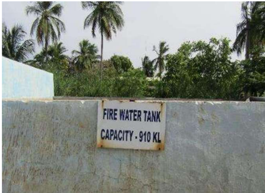
Dedicated Water Reservoir Capacity – 910 KL
