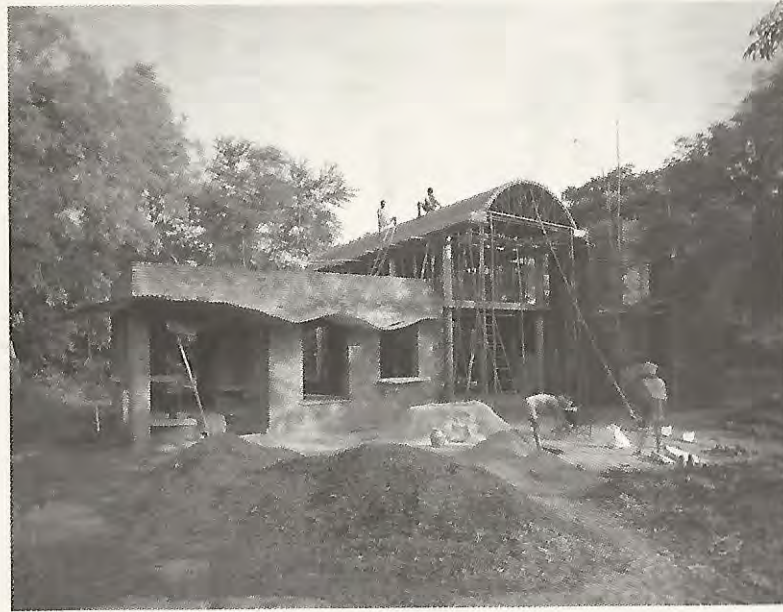
Building a new house
