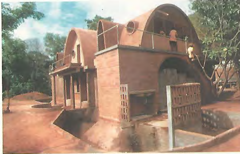
Earth block construction
