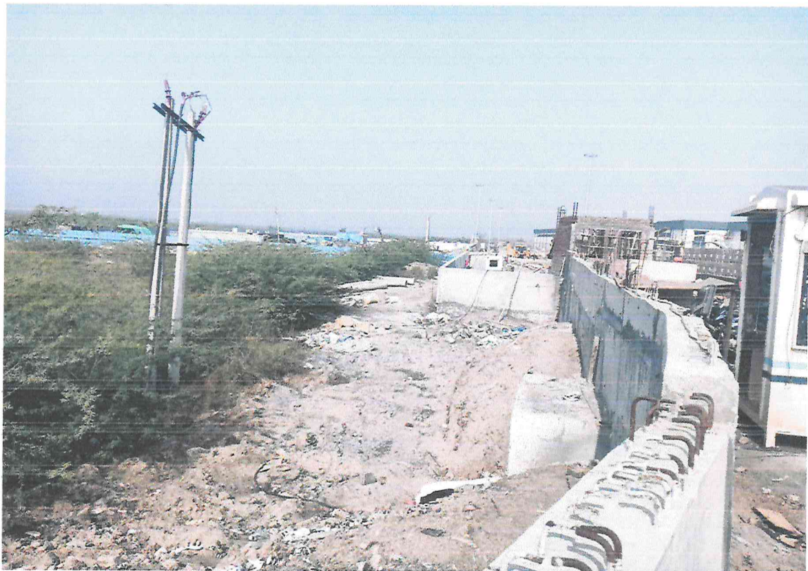
Picture 7: Grew Energy Pvt. Ltd., Kh. No. 1657, Bhojpur Road.
