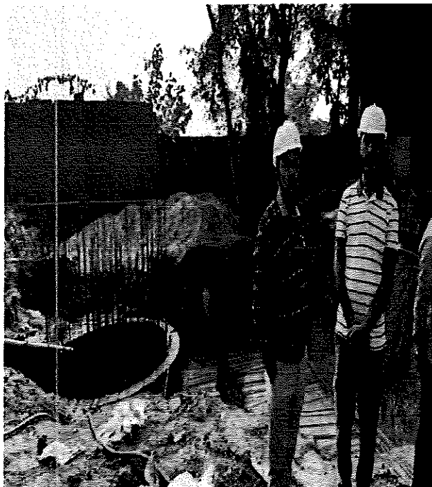
Photo 24: Photograph of Civil Work for installation of Stack
