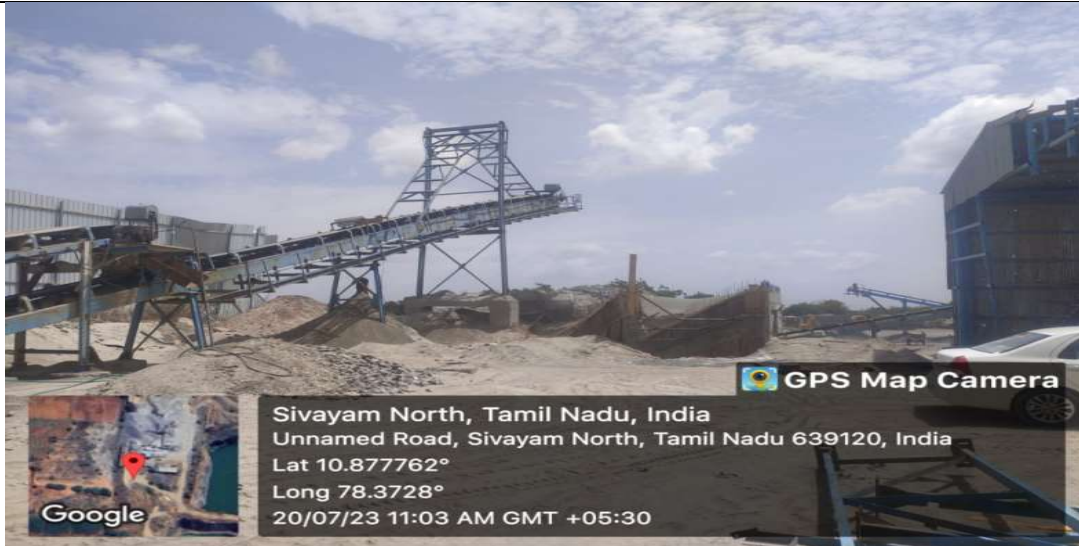
Conveyor removed connecting primary crusher and secondary crusher
