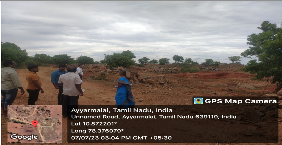
Preparatory work for quarry site under progress.
