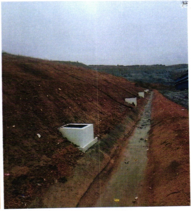
Above are separate sumps for collection of legacy leachate generated from capped dump. The leachate collected in these sumps is either pumped or transported through tanker to the below integrated collection sump for storage before treatment.
