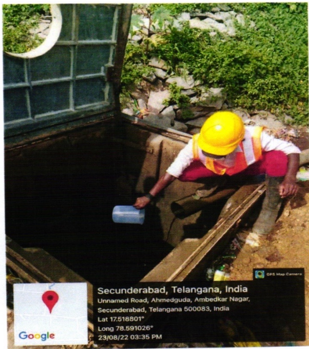
Above are separate sumps for collection of legacy leachate generated from capped dump. The leachate collected in these sumps is either pumped or transported through tanker to the below integrated collection sump for storage before treatment.
