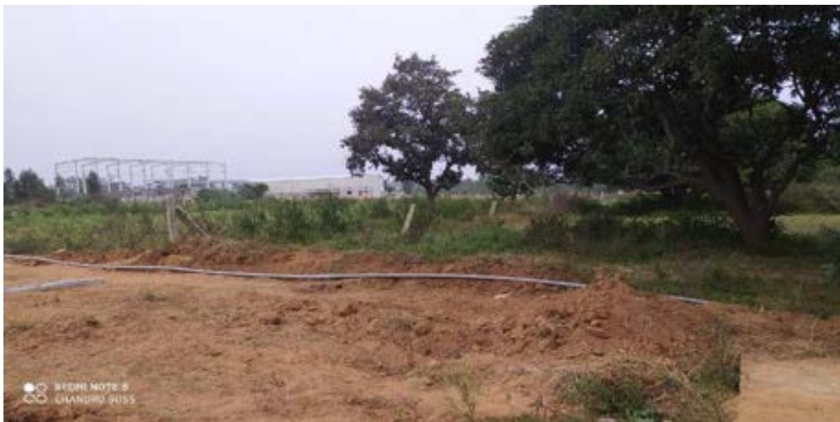
Survey work, Barbed Wire fence poles on all sides & building construction
