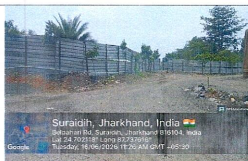
Fig. 18. Tin sheet boundary wall
