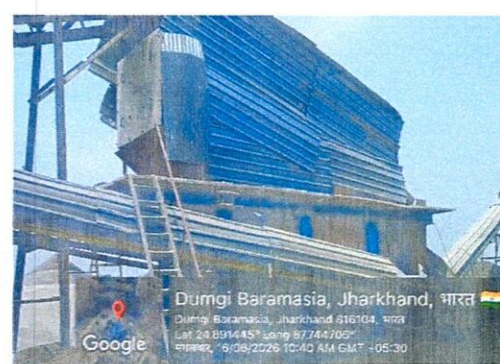
Fig. 24. Crusher Screen and conveyor belts are covered with tin sheet.
