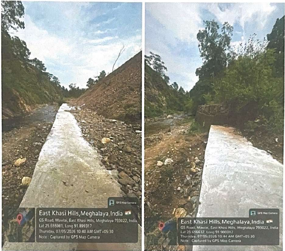
The two Retaining walls that have been constructed
