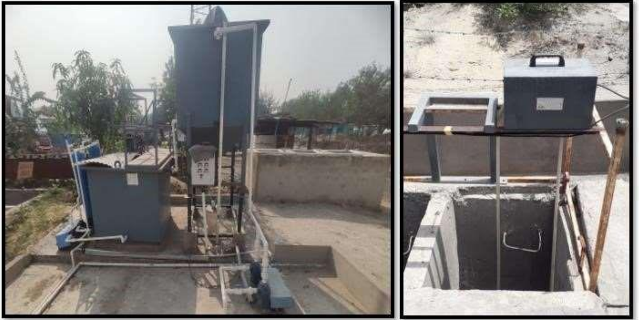
Fig 04- State of the art ETP in working condition with Oil Skimmer
