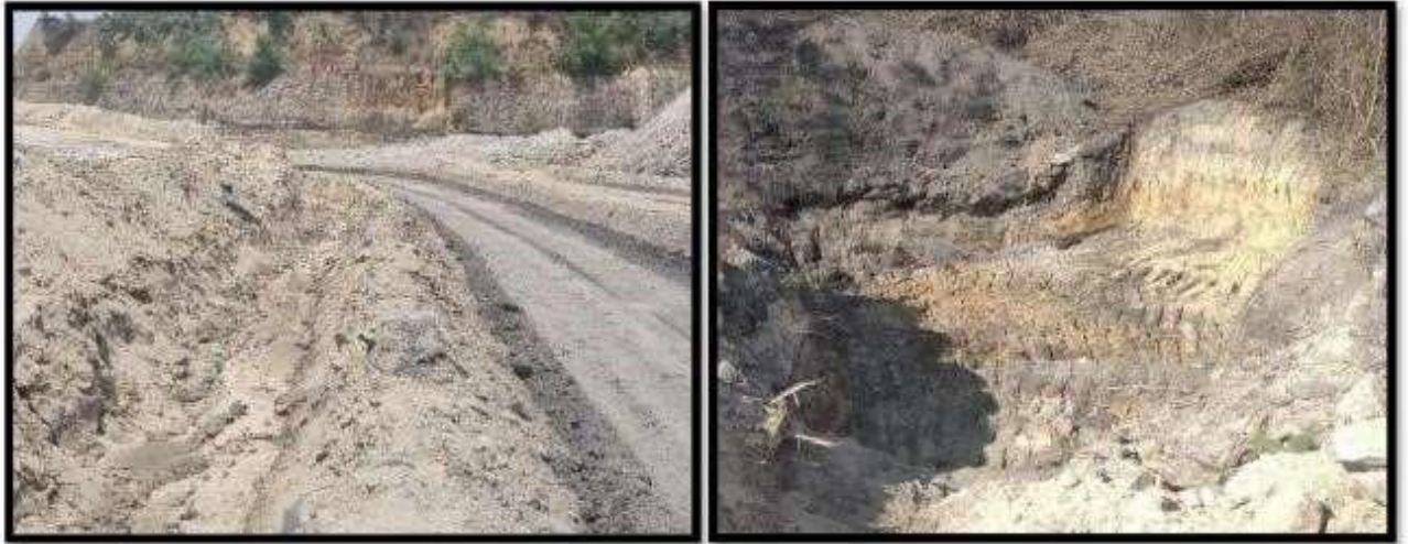
Fig 2- Garland Drain and Siltation Pond
