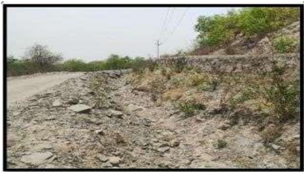
Fig 8 – Toe Wall along the Dump
