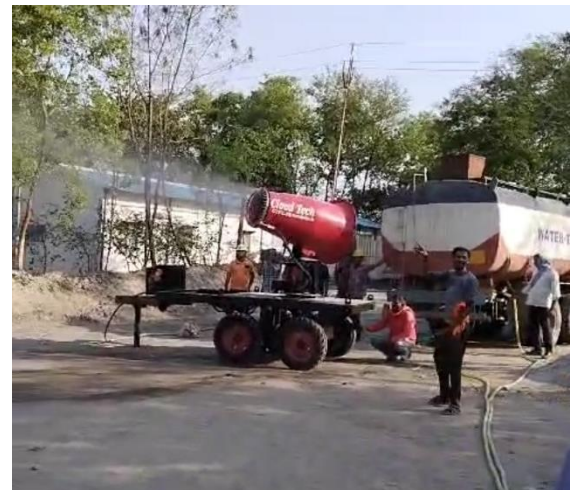
Fig 05- Fixed Type Water Sprinkler along Haul Road and Fog canon in Coal stock
