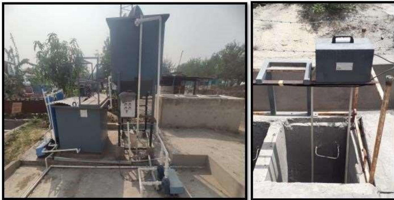
Fig 06- State of the art ETP in working condition with Oil Skimmer
