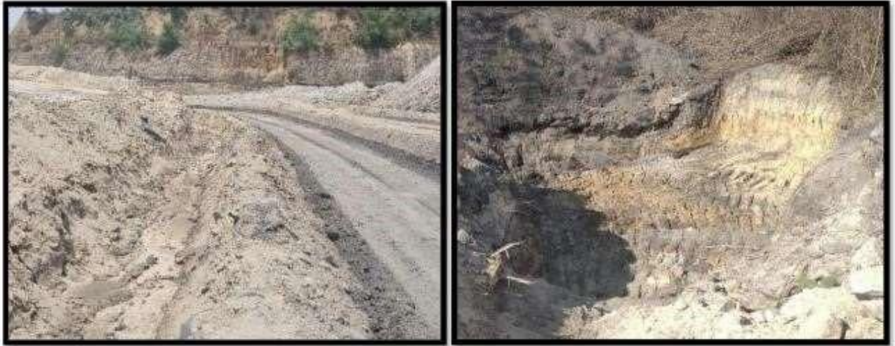
Fig 2- Garland Drain and Siltation Pond
