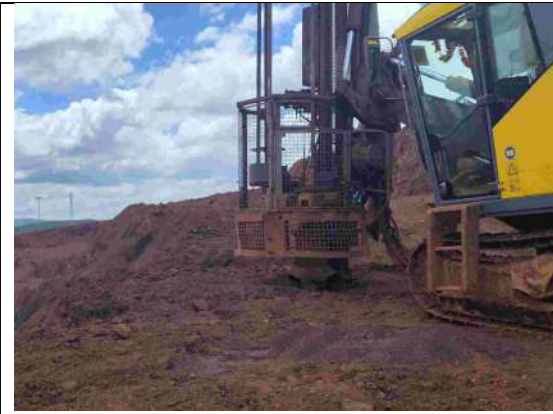
Photo 15: Wet drill machine
