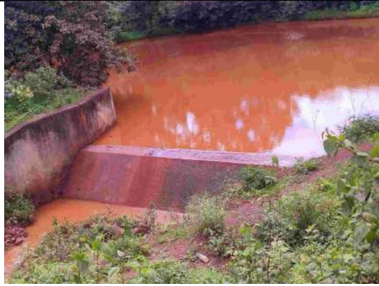
Photo 8: Check dam on seasonal nala
