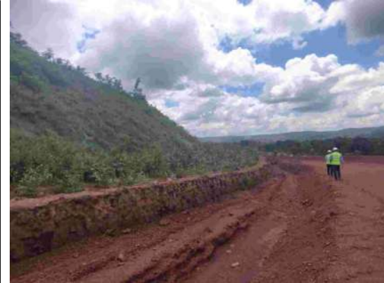
Photo 17: Toe wall and garland drain
