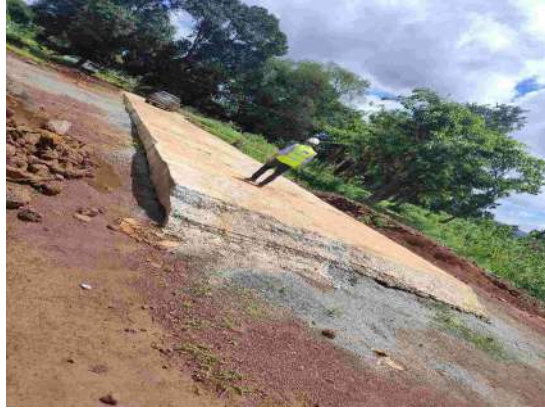
Photo 10: Concrete road to Mn Quency
