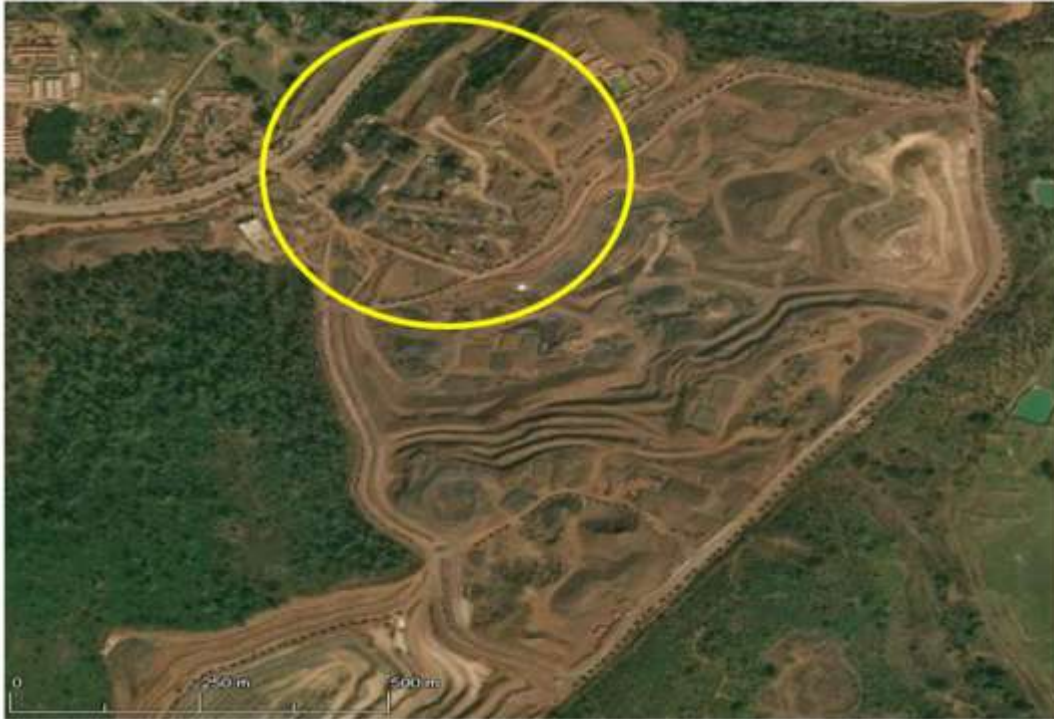
[Construction of 6MTPA iron ore beneficiation plant by JSW at Narayanposhi mine in 2023.]
