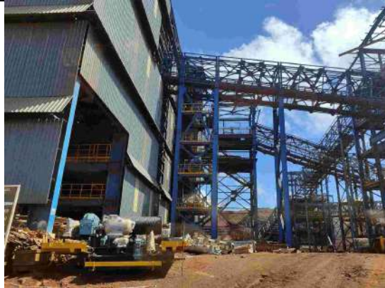
Photo 4: Under Costruction benficiation plant
