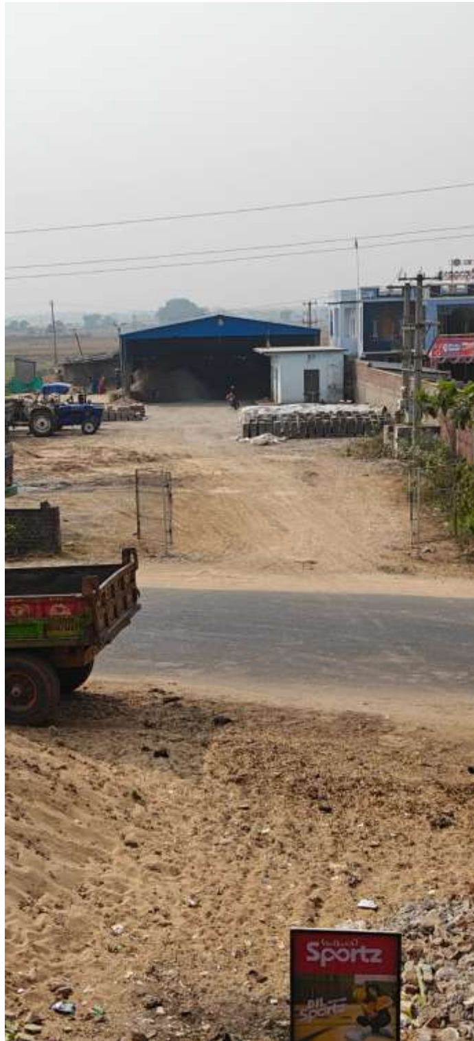
Fig:- Geotagged photographs of M/S Sadhu Baba Bricks, located in Odei, near Jhumpuri Bazar, Po- Dasarathpur, Jajpur District: Fly Ash Manufacturing Unit's installed machinery, raw material storage, and present dust suppression measures.
