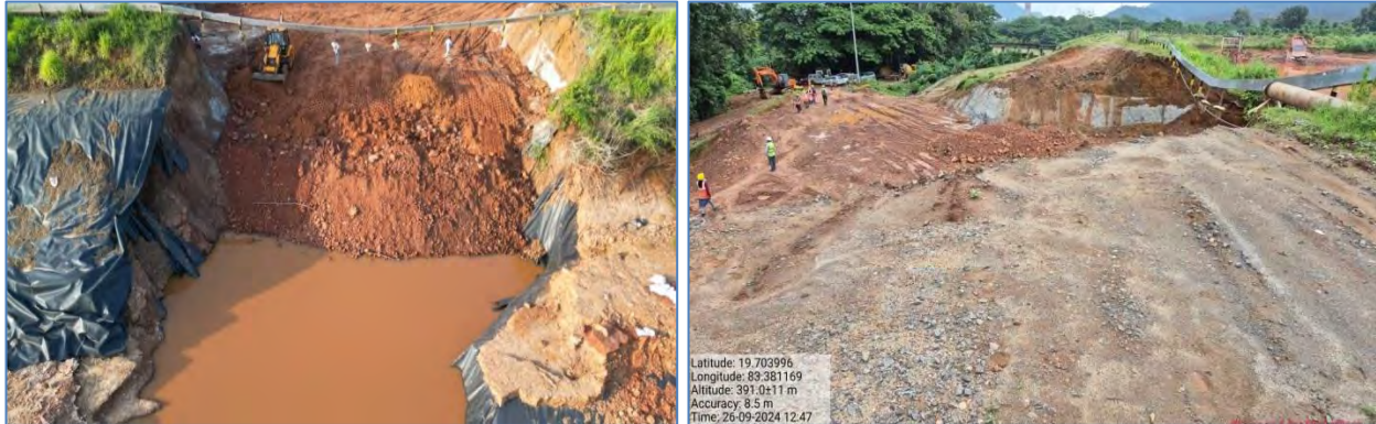
Figure-12 : Dyke Repair
