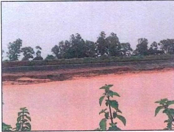
Fig. 2c: High water level mark on the upstream side of north dyke due to heavy rainfall
