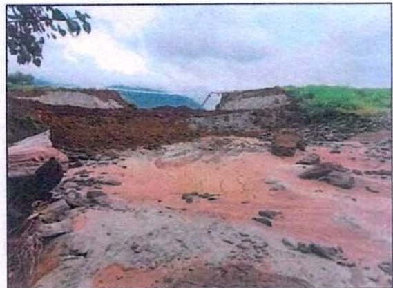
Fig. 2b: Temporarily closing of breach with locally available soil
