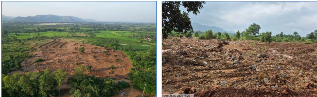
Figure-11 : Top Soil replacement of affected land with Fertile Soil
