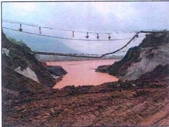
Fig. 2a: Dyke breach area
