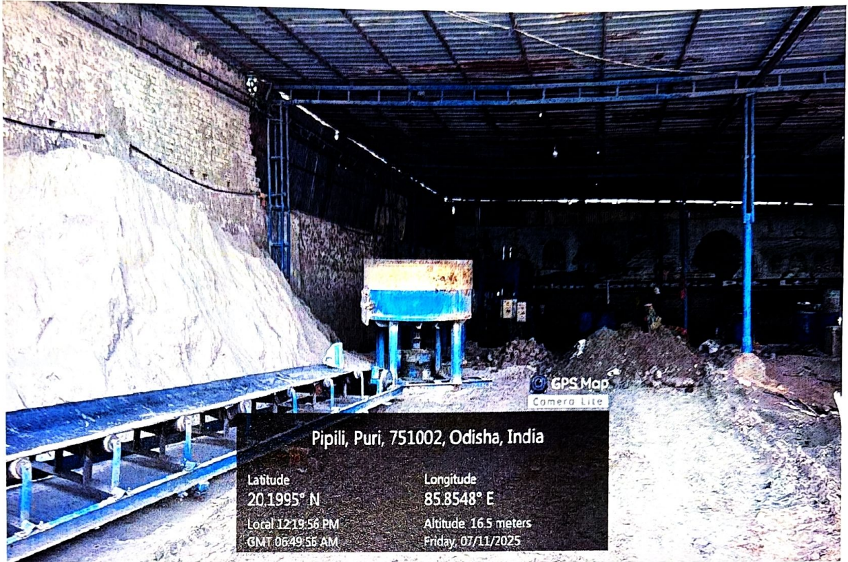
Raw materials storage and production process takes place under a common shed
