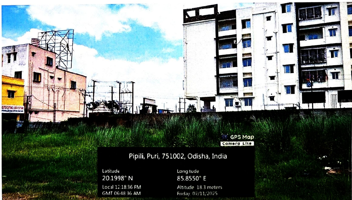
The factory and residential apartment separated by boundary wall
