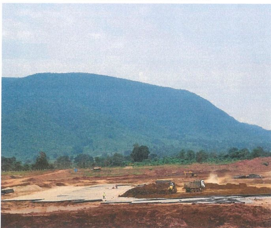
Soil overburden on HDPE liner
