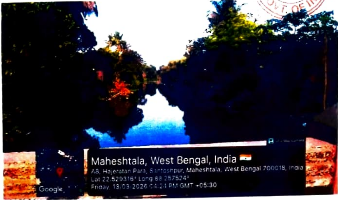
CH. 5810.00 M OF NEW MONIKHALI KHAL D/S OF SATGHARA RCC BRIDGE
