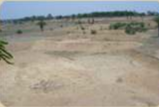
Rainwater harvesting structures
