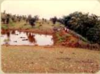
Drainage line treatment
