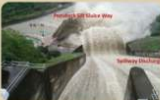
Simultaneous operation of spillway and penstock sluice venting turbid density current
