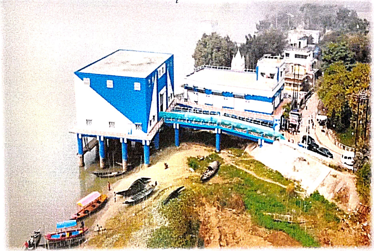
187 MLD INTAKE STRUCTURE COMPLETED
