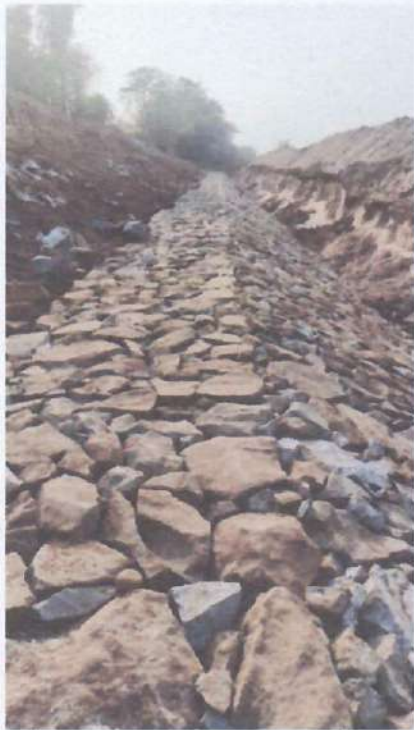
Bank protection by launching & Packing in right Bank of river Subarnarekha near village Dhitpura
