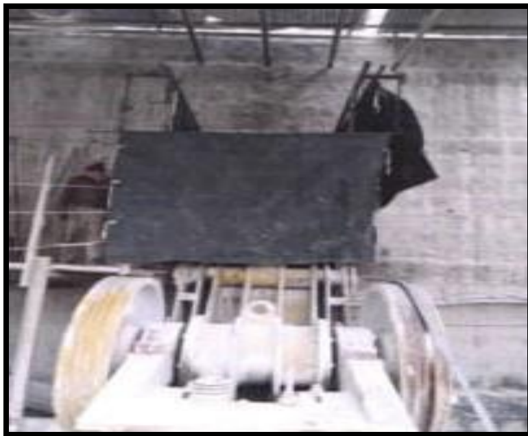
Figure-1: Covering of Primary/Jaw crusher
