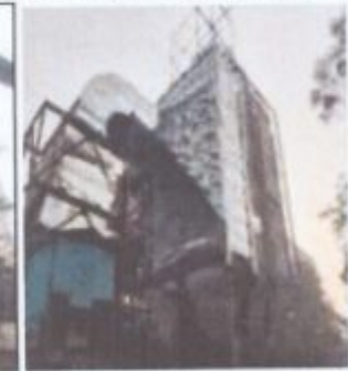
ESP of pellet plant
