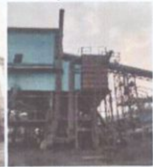
Coal Crusher Bag filter
