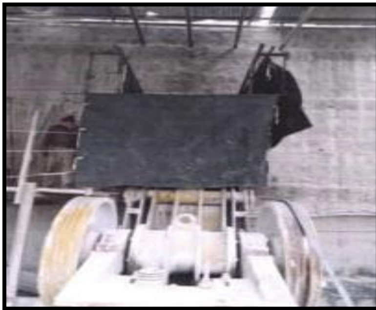
Figure-1: Covering of Primary/Jaw crusher
