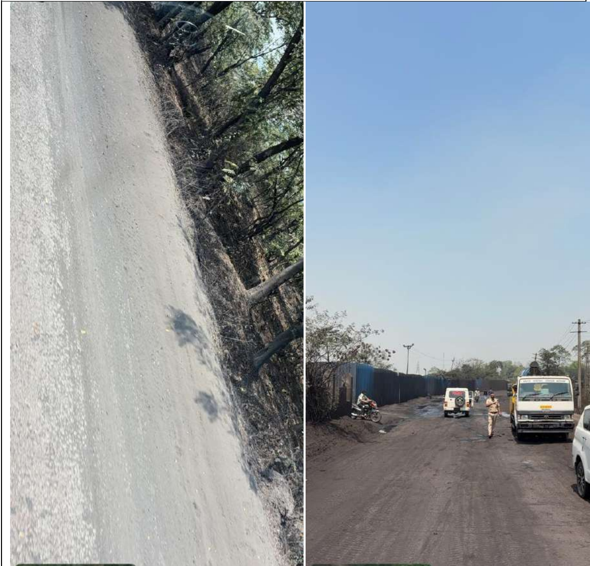
Dust accumulation on sides of road
