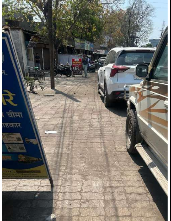
Road Shoulders Paved but not cleaned
