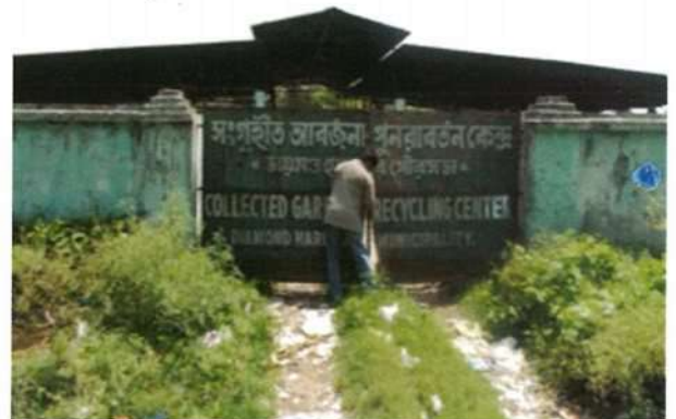
Material recovery facility at Diamond Harbour Municipality
