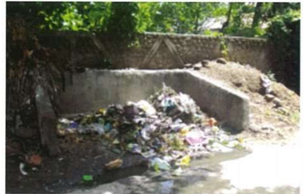
Masonry enclosure for dumping waste at local level at Tamralipta (Tamluk) Municipality
