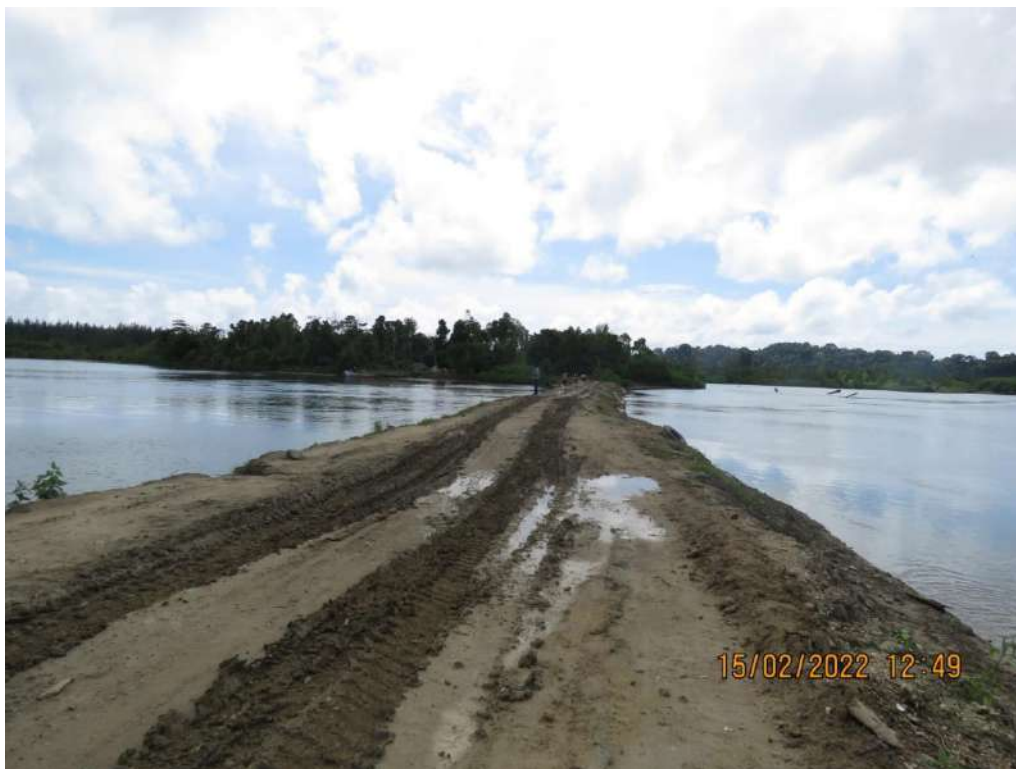
Plate 12: Road under construction by GRIF
