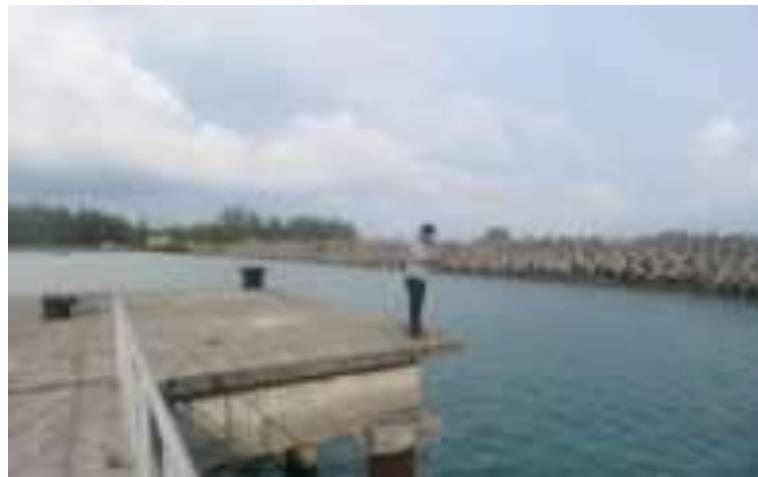
Another view of breakwater at Campbell Bay
