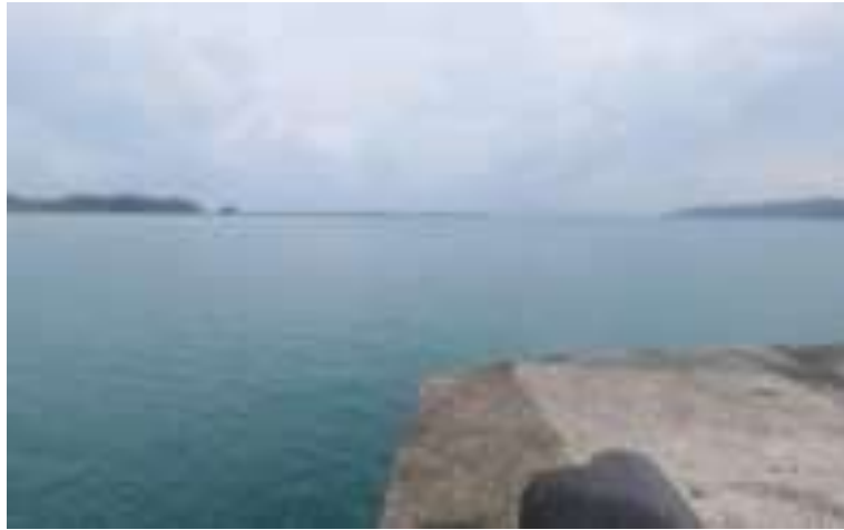
Another view of breakwater at Campbell Bay
