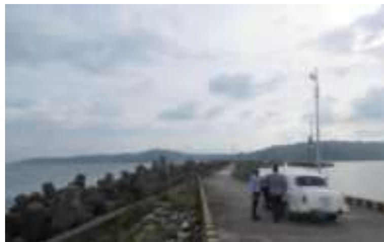
View of breakwater at Campbell Bay
