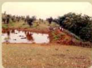
Drainage line treatment
