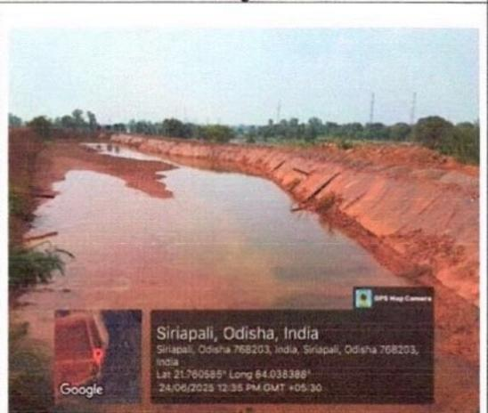
Decantation pond of Iron ore tailing pond-2 with HDPE liner
