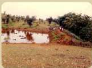
Drainage line treatment
