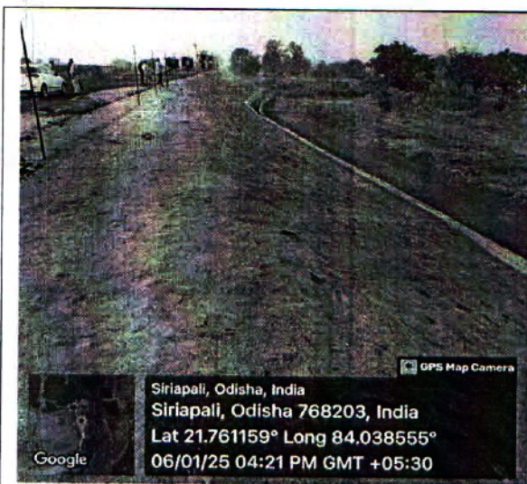
Stone pitching work of the Tailing Pond towards the village Bisadihi
