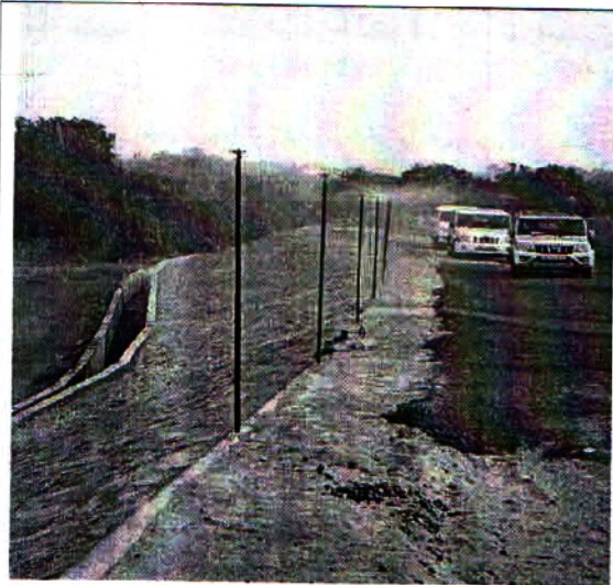
Fixed type water sprinklers around the Tailing Pond No. 2 & 5 in operation
