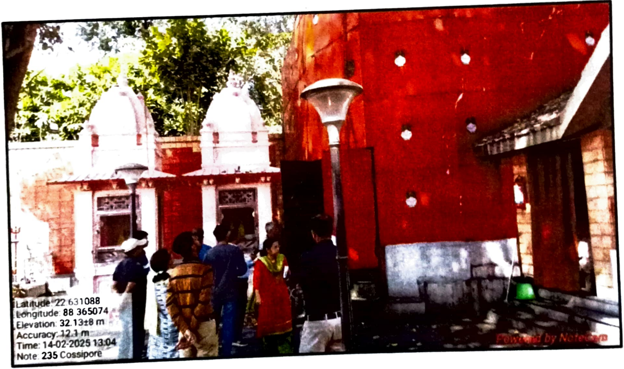
Inspection at Sri Sri Ramkrishna Mahasamsan Burning Ghat
