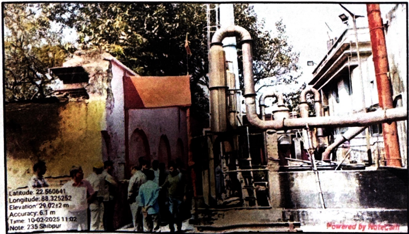
Inspection at Shibpur Burning Ghat
