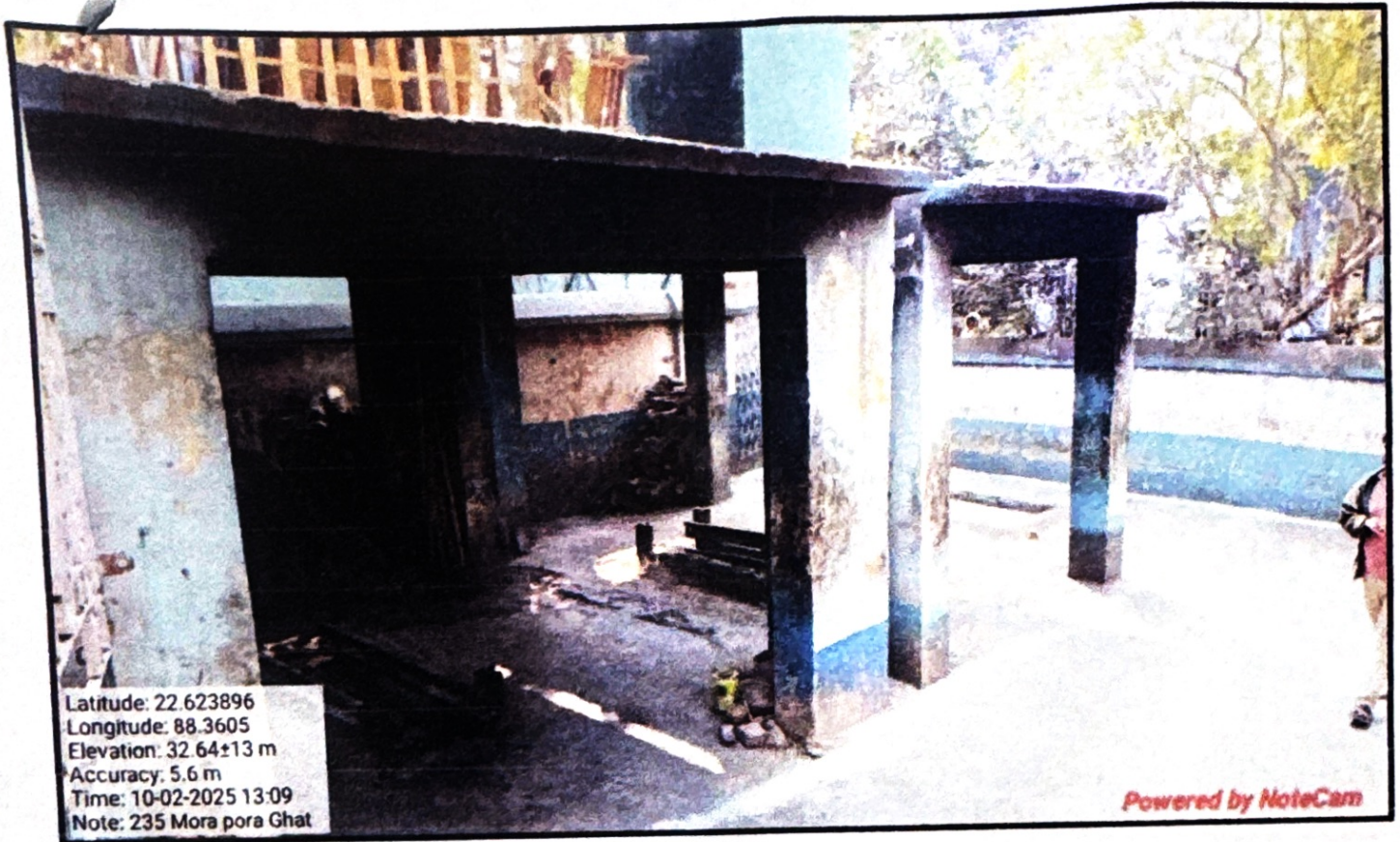
Inspection at Morapora Burning Ghat
