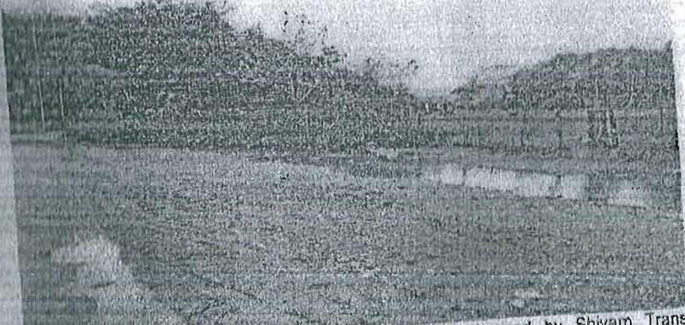
Picture:7: The raised level of the river bed due to mixing RBM with of muck/debris dumped by Shivam Trans Construction Private Limited. The raised level of river bed has changed the course of the river, letting them into the paddy fields of the local poor people.
