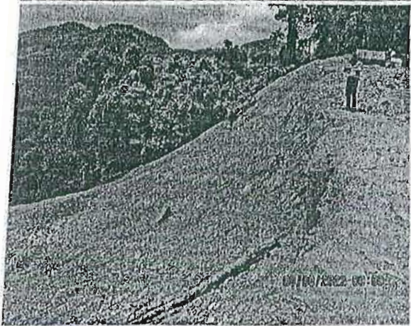
Photo 1&2. Mucks disposal nearby waterbody and natural vegetation and not maintained the slope.
