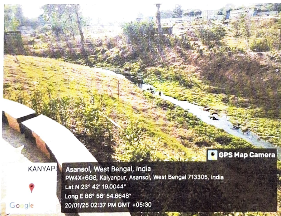
Pic.3: Major drain flowing through the Shristinagar complex
