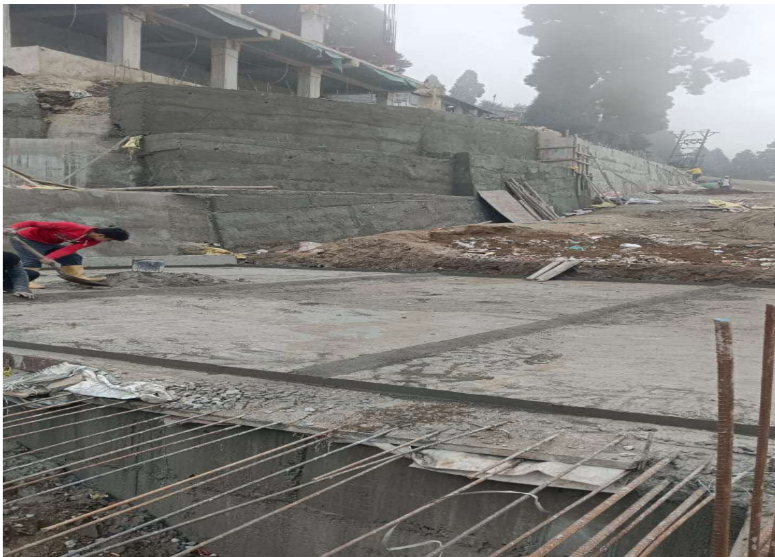
CONSTRUCTION OF MULTI CELL RCC CULVERT FOR SWM PROJECT
