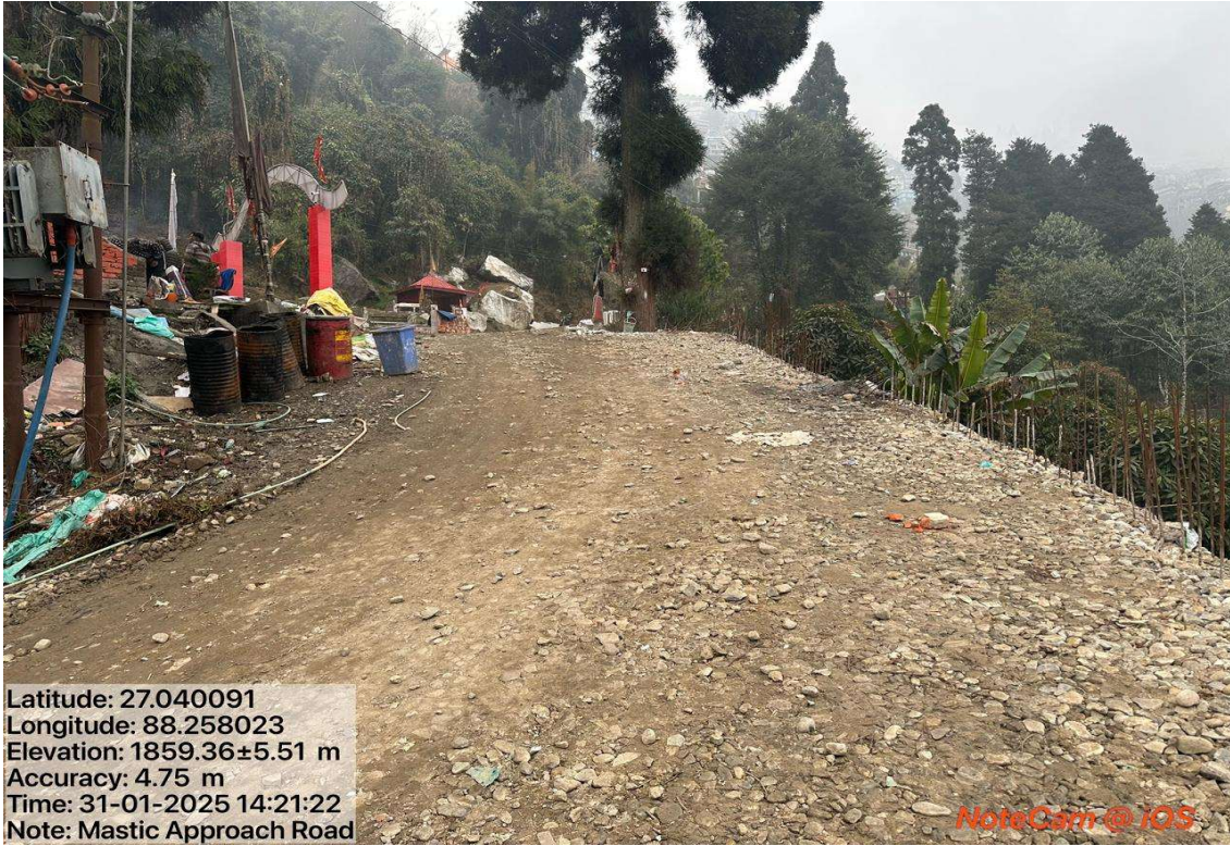
BITUMINOUS MACADAM WITH MASTIC ASPHALT APPROACH ROAD
